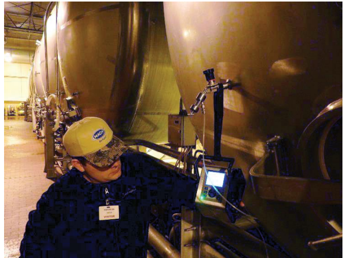
Figure 4: Portable Orbisphere 3100 used for on-line verification
